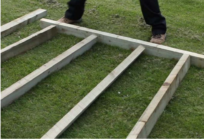
An 8 x 6 Portabase laid out on flat ground ready to assemble.
