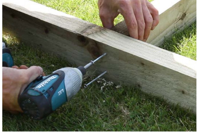
Screw the frame together.
